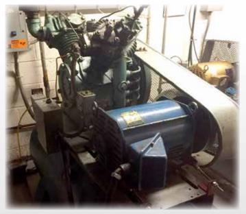
"Another benefit (provided by LE) is the LEAP<sup>™</sup> oil analysis program. We had a high metal flag on a sample. Inspection found bearing journal wear on one shaft. We had time to procure and install a new gearbox without an hour of downtime."
